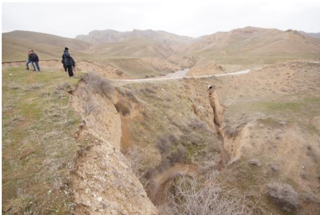
Plate 9: The erosion gully formed, and aggravated by the culvert
