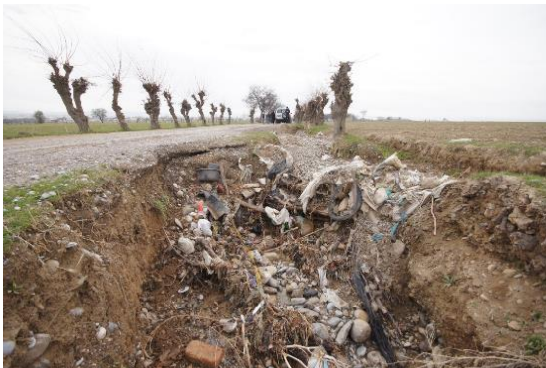
Plate 5. Erosion due to the runoff, threatening the road; garbage management issue.
