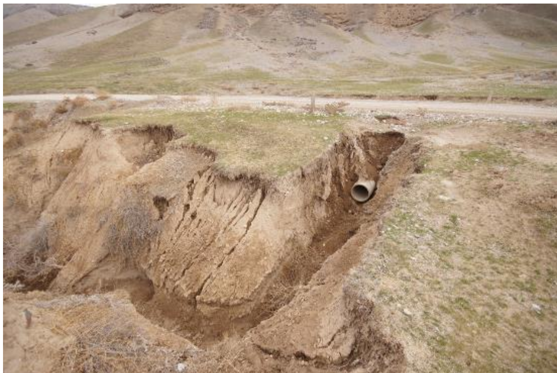
Plate 6. Gullies triggered by the culvert
