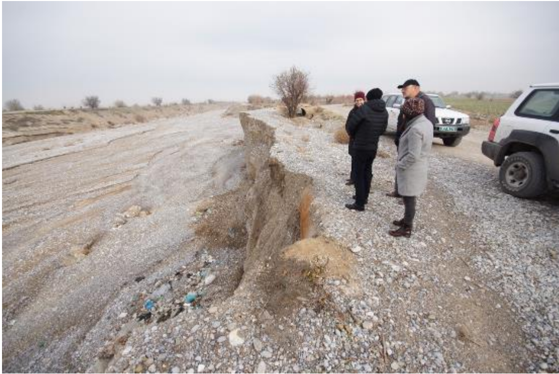
Plate 3: the external bend of the river, 8m above the canal. Observe the buried (rusty) pipeline linking two portions of the irrigation canal at the feet of the team, on right bank. On the left bank (the inside of the bend), some concrete slabs remain.
