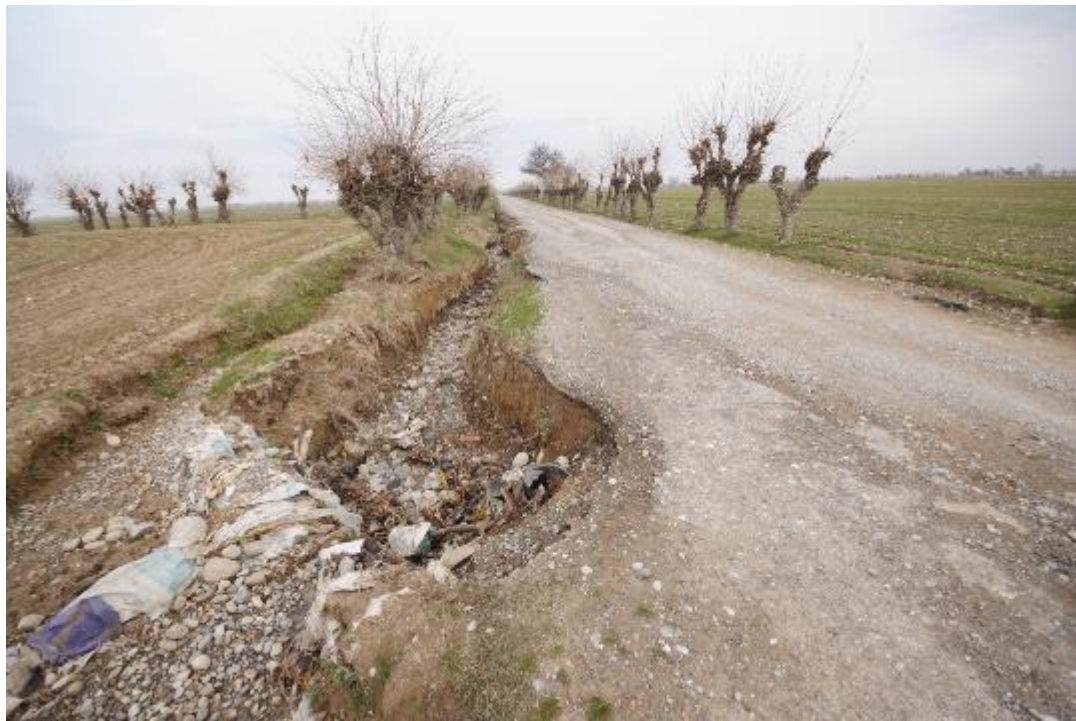
Plate 4. Erosion due to the runoff, threatening the stability of the road, and the fields
