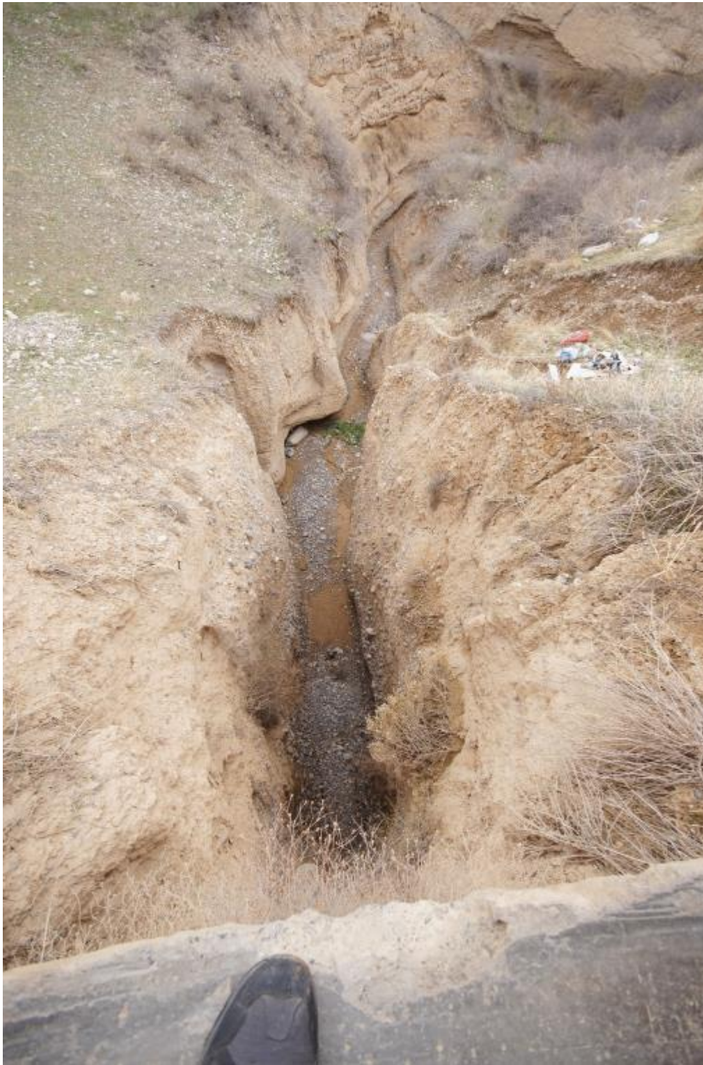
Plate 10. The erosion gully seen from inside the culvert (height: approximately 10m)
