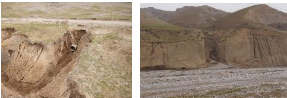
Figure 4: pictures from field trip. Left: erosion after drainage pipe below a road. Right: huge erosion gully leading into Isfana river.
